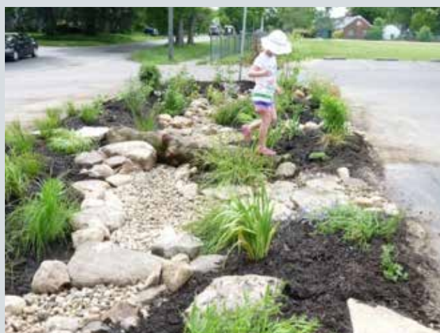
FIGURE 3.8: Examples of bioretention cells and rain gardens (images courtesy of centralohioraingardens.org )
