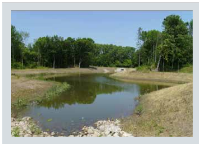
FIGURE 3.5: Example of an “online” regional detention pond, although they typically have more vegetation (image courtesy of rvtcorp.com)
