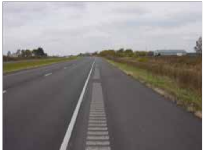
FIGURE 3.4: Paved shoulders allow bicycles to safely travel on a rural roadway without impeding traffic along the corridor. Maintain adequate distances between higher speed traffic and the bicycle will also increase the comfort level of the bicyclist.
