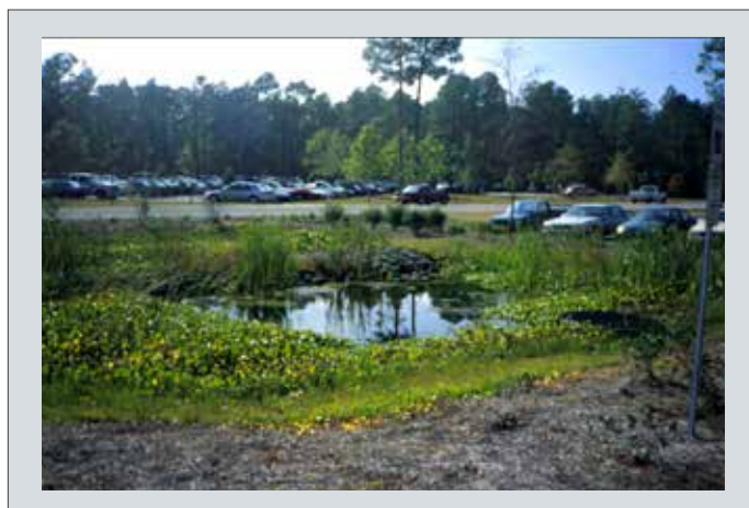
FIGURE 3.6: Small constructed wetland for stormwater detention and water quality improvement (image courtesy of uncw.edu)
