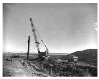
**Figure 6.**LS-98 Link-Belt Speeder Crane Preparing Bridge Footing for I-80 Bridge Near Bettendorf dated 1-10-1957. (Courtesy of Iowa Department of Transportation, Photo Id. HA1.050.0030)
