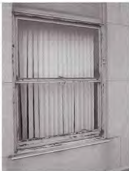
Fig. 2. View of an unrepaired steel-framed window on the east elevation of the Lafayette Building. Note the loss of paint coatings and corrosion of the built-up steel frame.
