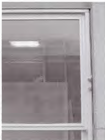
Fig. 7. Head of the repaired window. Note the similar sight lines but missing articulations and accessories of the replacement window when viewed in conjunction with the repaired window.
