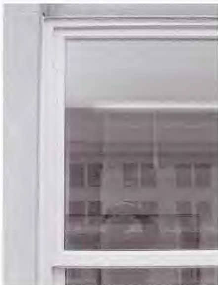
Fig. 6. Head of the replacement window.
