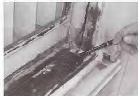
Fig. 3. View of a steel window sill on the east elevation of the eleventh floor. Note the significant corrosion of the steel frame at the sill-to-jamb corner.
