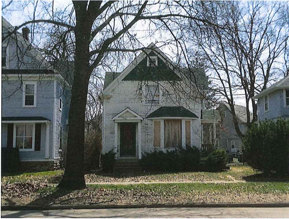
Picture #1 Front View (West)
