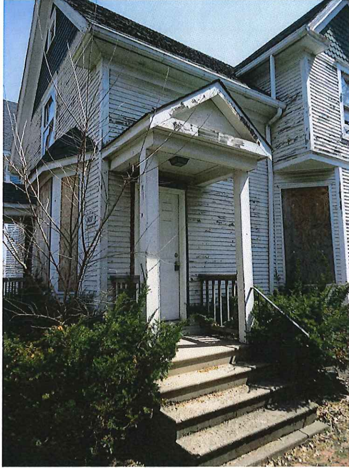
Picture #5 Side Porch & Door
