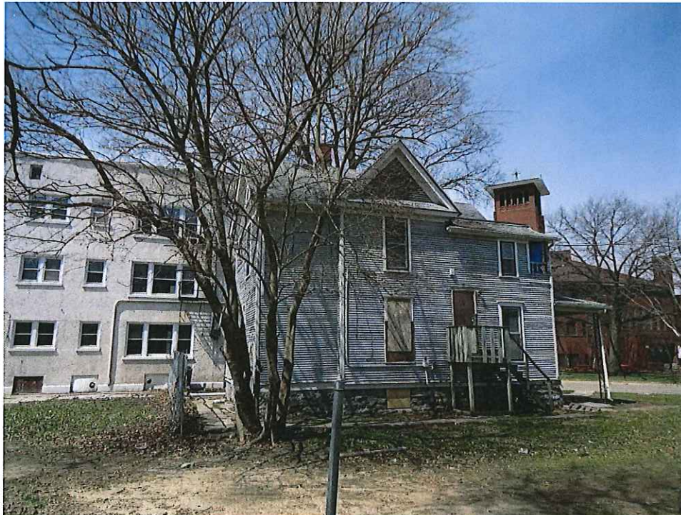
Picture #2 Side View (East)
