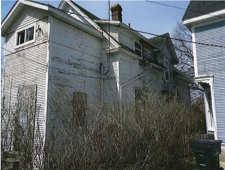
Picture #2 Side View (North)
