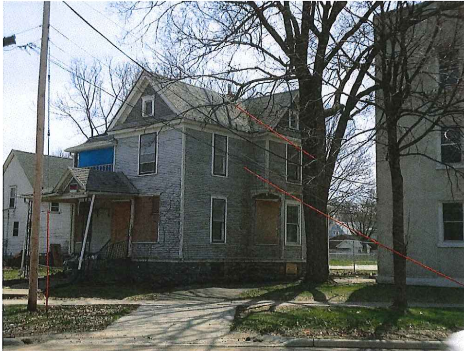
Picture #4 Side View (West)
